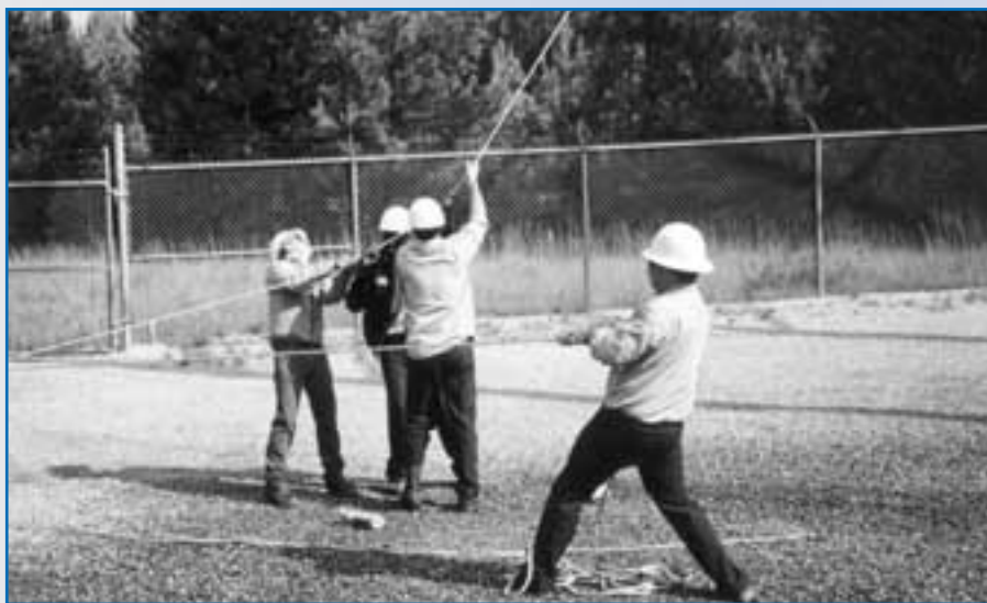
Line Technicians hoist heavy insulators up to Technicians working on the pole.
