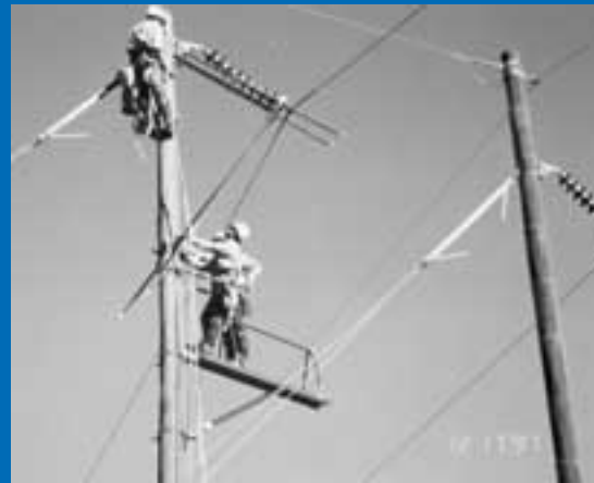
Line Technicians changing out suspension bell insulators on 138,000 Volt transmission line.
