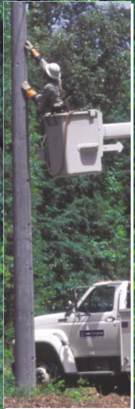
Sam Houston EC's Right-of-Way Program is a continuous, preventative maintenance schedule of trimming trees, removing dead trees and mowing underbrush.
