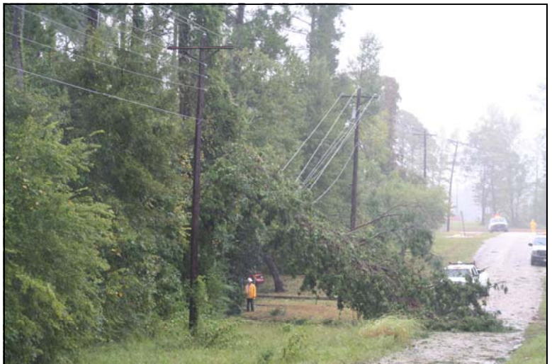
Right-of-way crews remove trees from lines near Coldspring Saturday.
